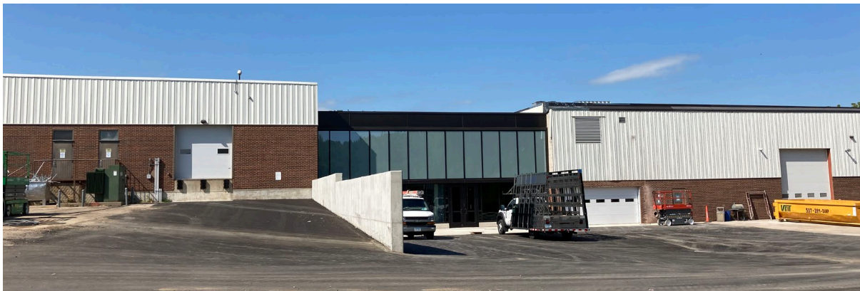
Figure 2: Image of new in-fill addition at rear entry to building
