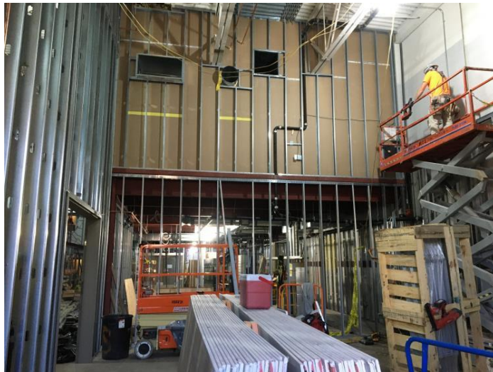
Figure 2 Wall Framing in Progress
